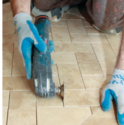
Multi-tools can be used for such tasks such as cutting out drywall (far left), removing grout and excess thinset (left), and trimming door jambs (below).
